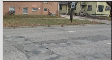
*Temporary patching of the failed asphalt surface*
